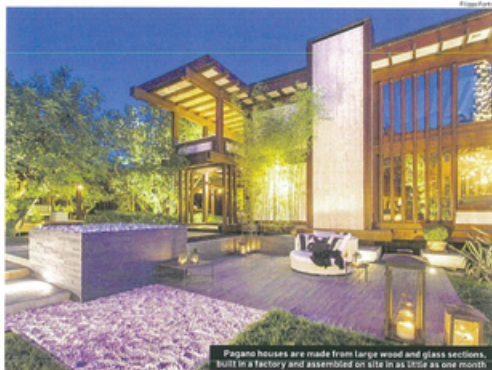
Pagano houses are made from large wood and glass sections, built in a factory and assembled on site in as little as one month.
